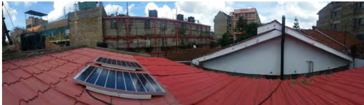
Figure 9: The 200W solar array on top of the 'kitchen laboratory' where the 'eCookBox' was installed.
