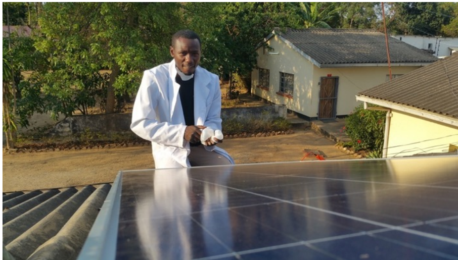
Figure 54: Bolting the PV onto the mounting frames.
