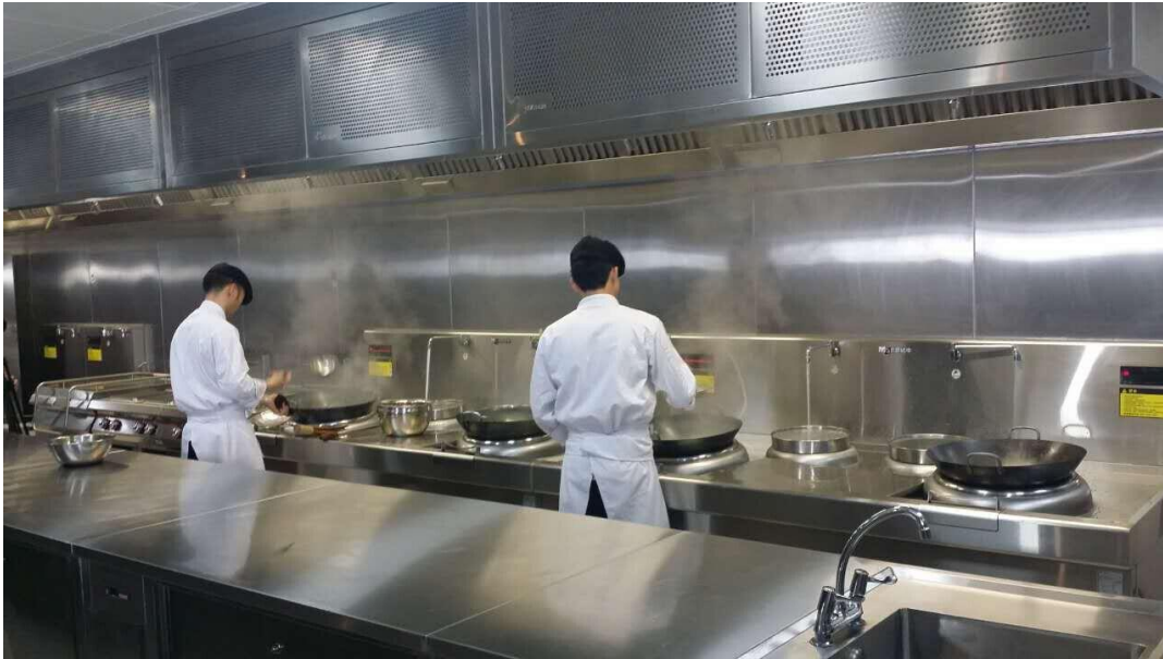
Figure 3: A typical 'All-electric kitchen' in China. The concave stovetop making sure full contact with the wok is in fashion.
