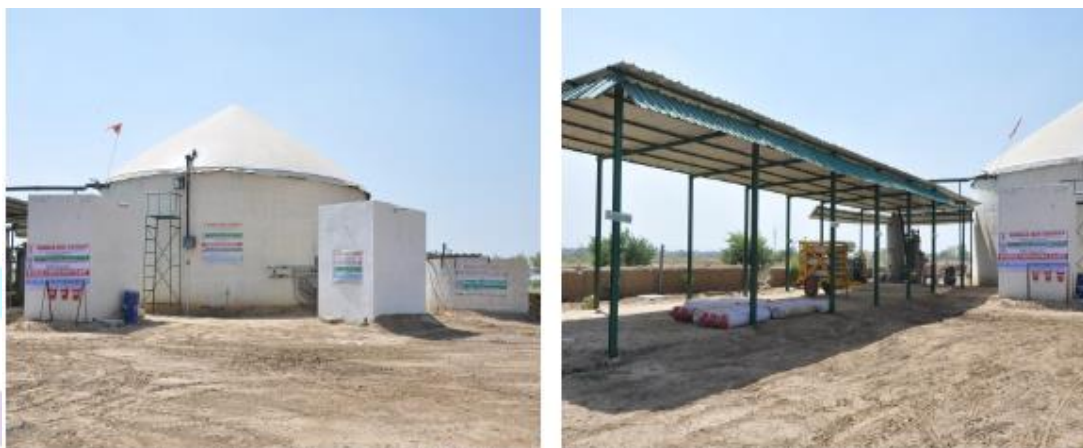
Biogas bottling project at Singla Bio-Energy, Vill.-Siaghawali, Teh.-Sadulsehar, Dist.-Sri Ganganagar (Rajasthan)
