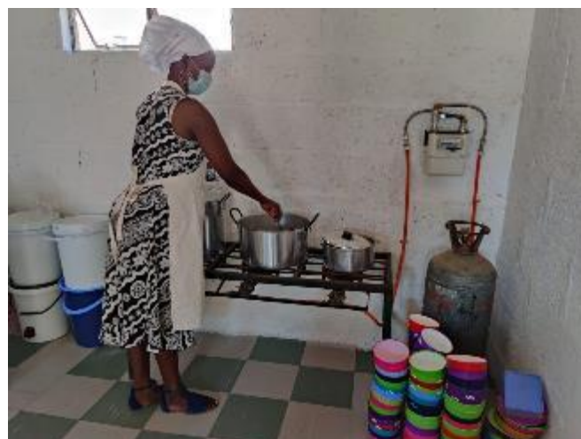
Figure 20 – Locally made LPG stove and cooking pots used for cooking school meals before EPCs introduction
