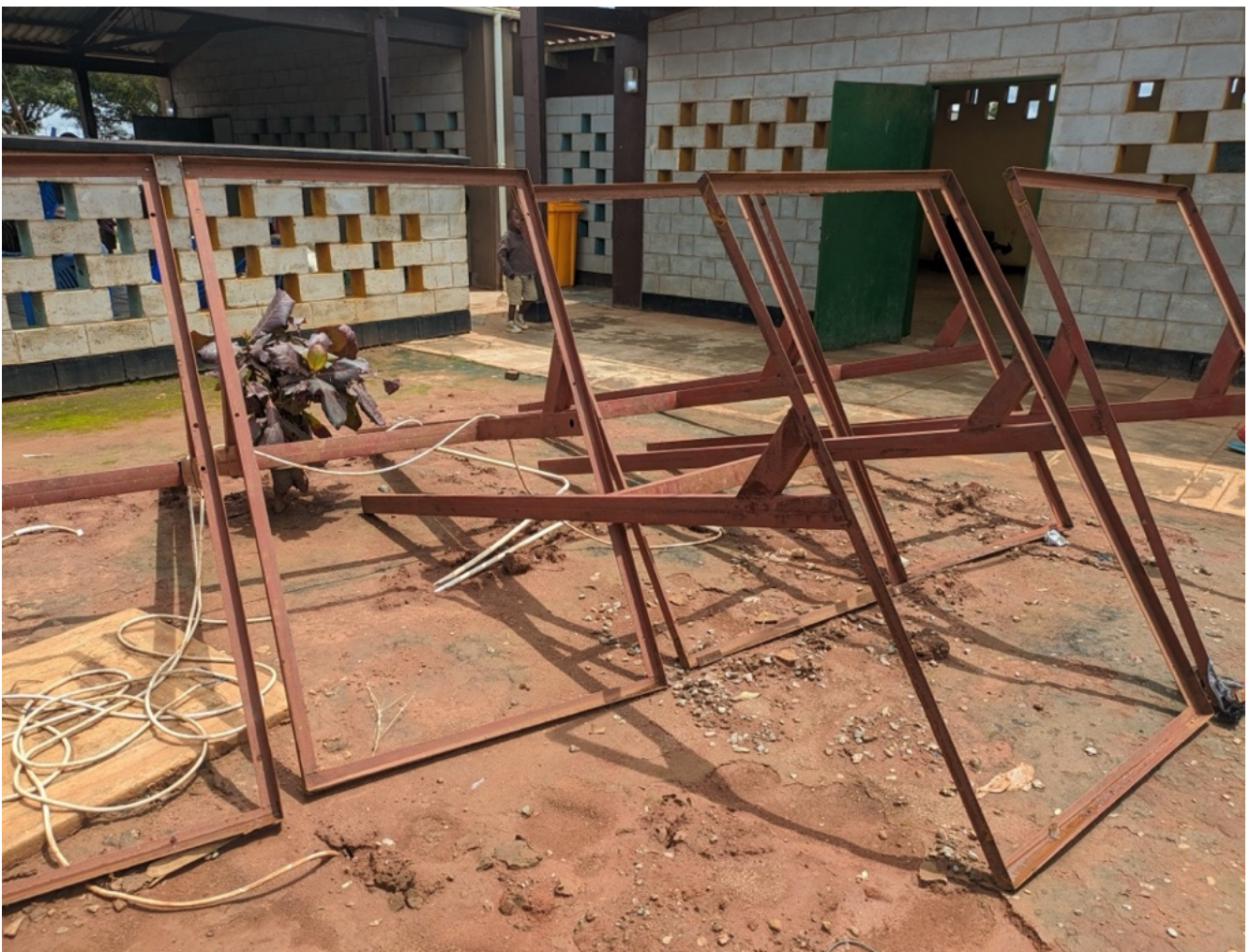
Image 17: Solar panel stands in Centre after removal of ECOCA (JFT, January 2024)
