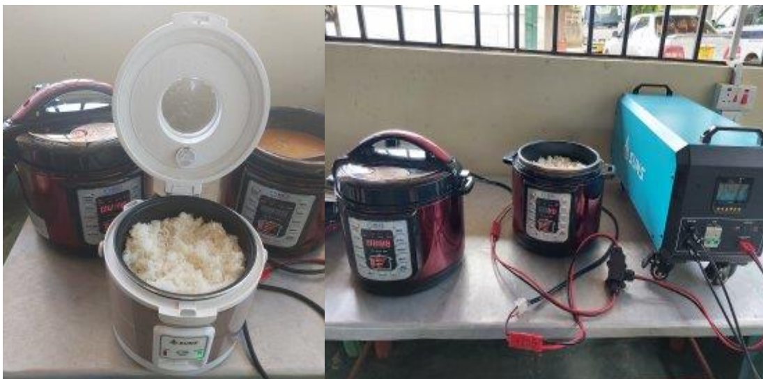
Testing of the systems after installing the monitoring devices.
