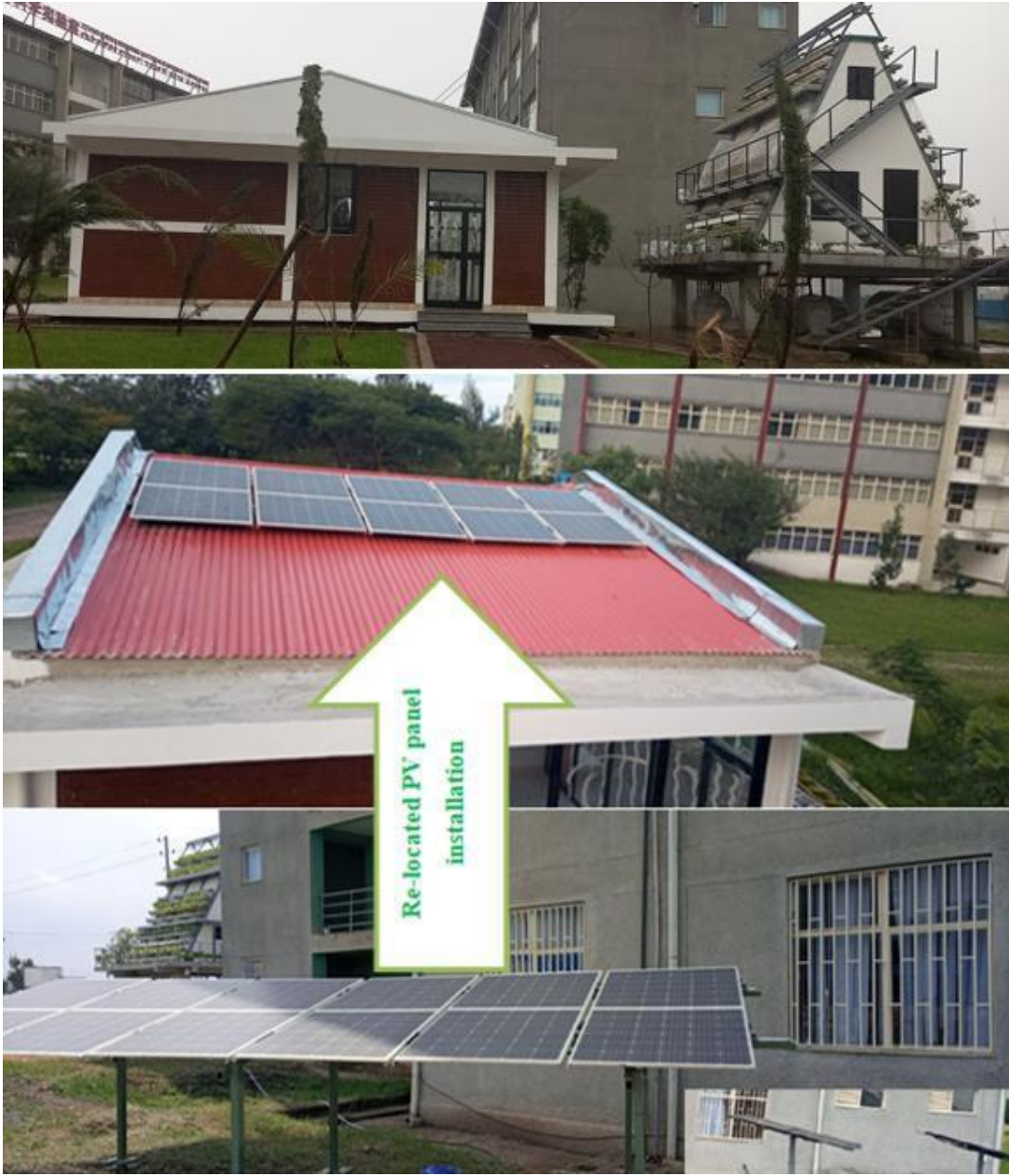
Figure 25: Repositioning PV panels on the purpose-built green lab house
