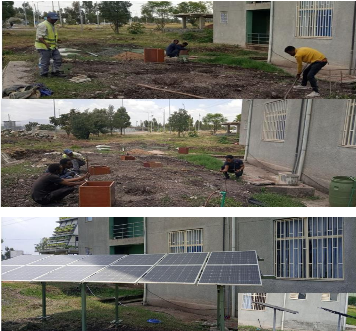
Figure 4: second phase PV panel installation accomplishment
