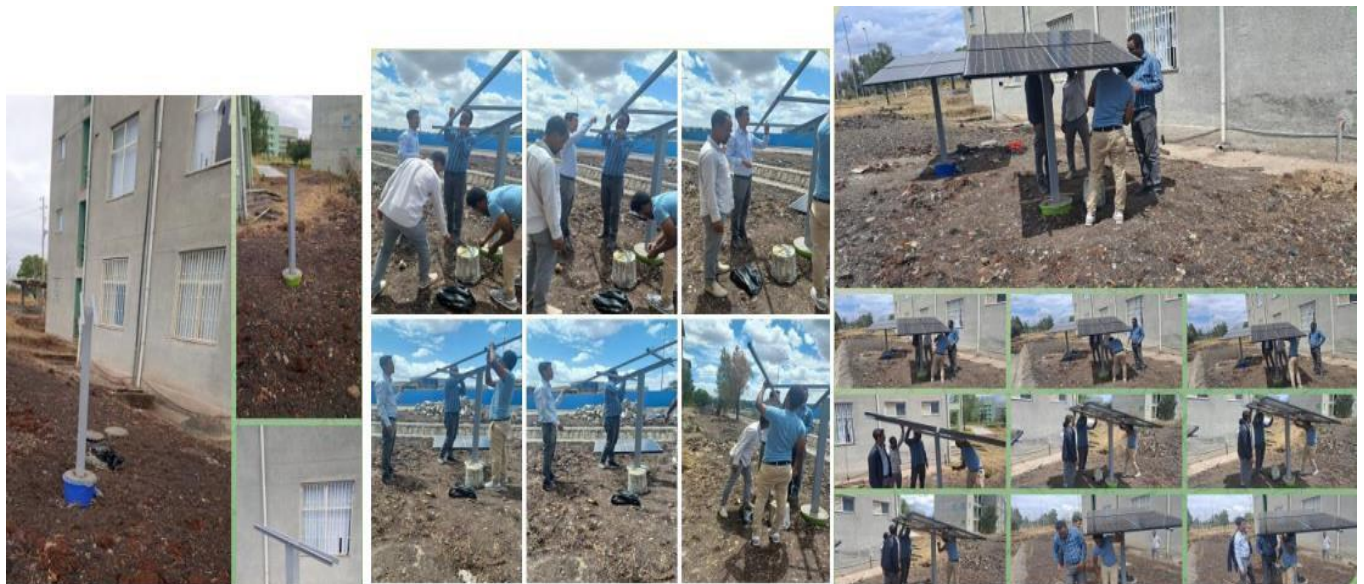
Figure 3: site work for PV panel installation
